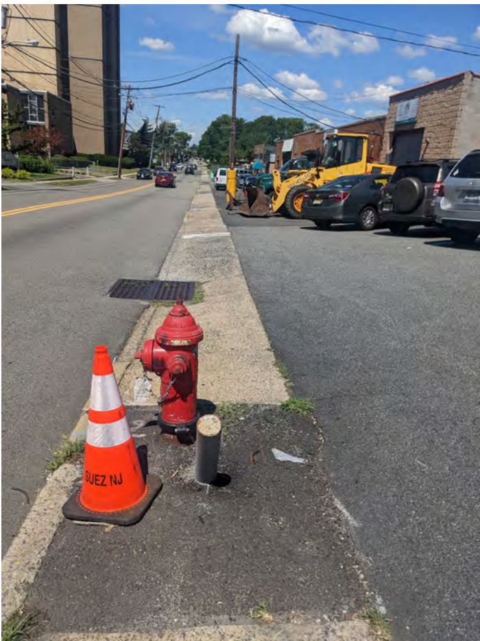
HYDRANT ALONG PROPERTY FRONTAGE OBSTRUCTING SIDEWALK AND VULNERABLE TO VEHICLES ENTERING AND EXITING THE SITE
