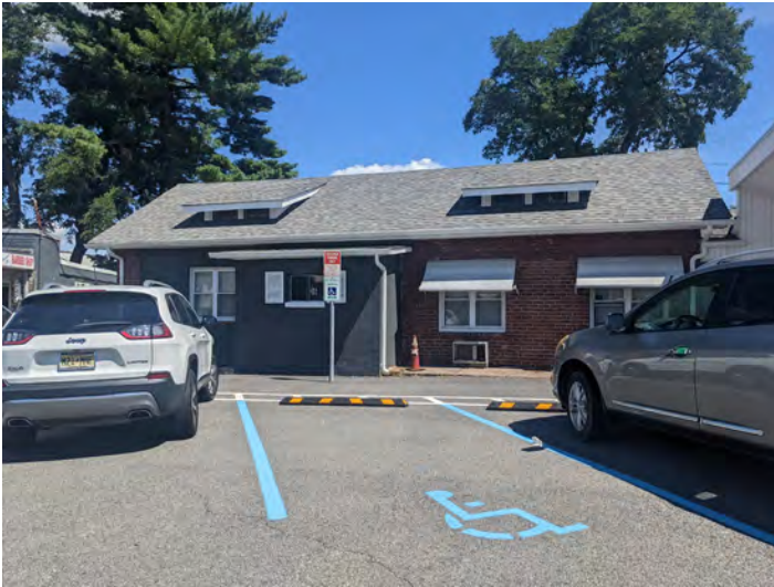
ADA SPACE WITHOUT ACCESS AISLE
