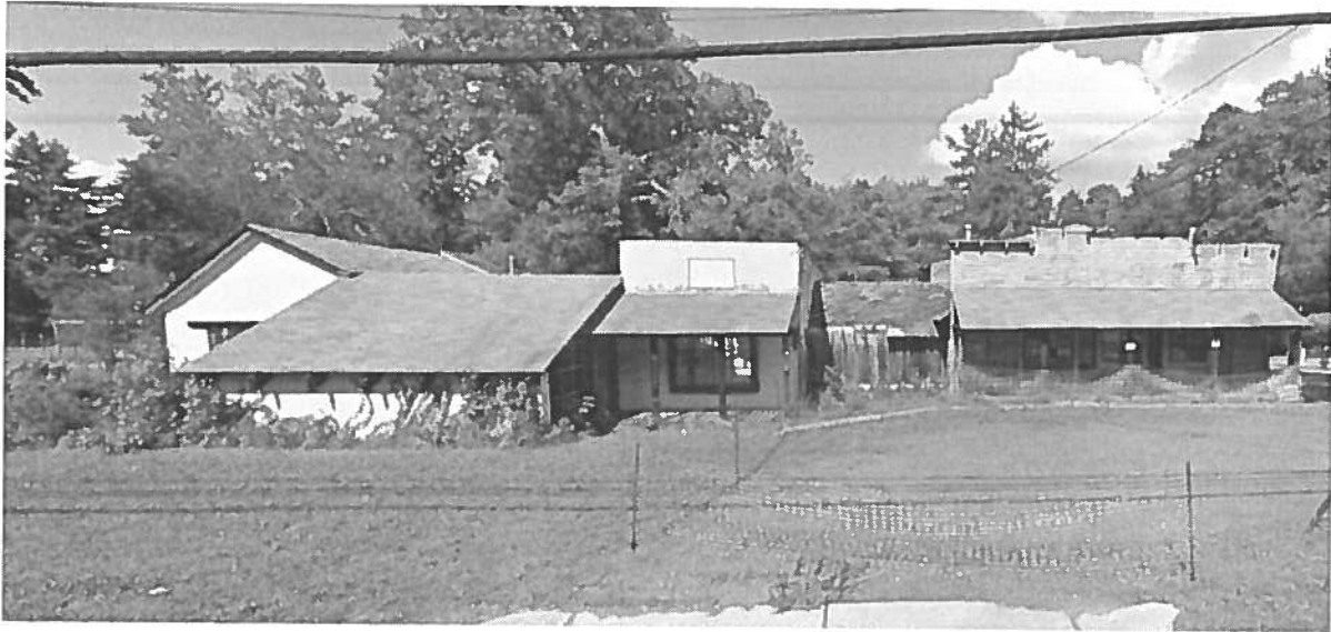
Prior to demolition:
