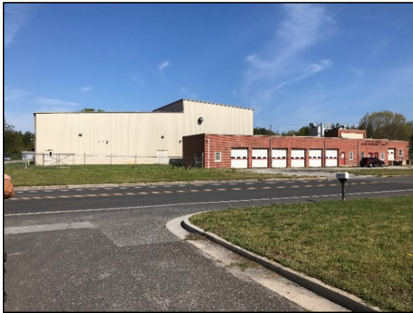
Water Treatment Facility
