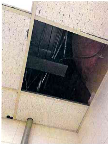
Plenum Area – Clean Steel Deck
