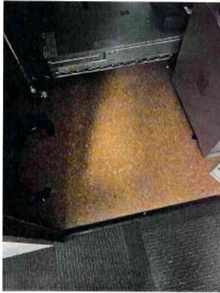
Storage Room Floor Tile
