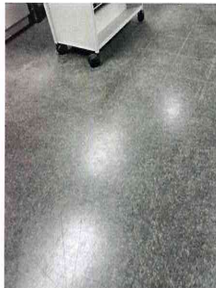
Circulation Office – Floor Tile
