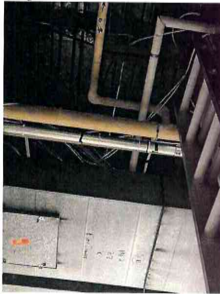
Overhead Pipes – Fiberglass Insulation with Solid Elbows
