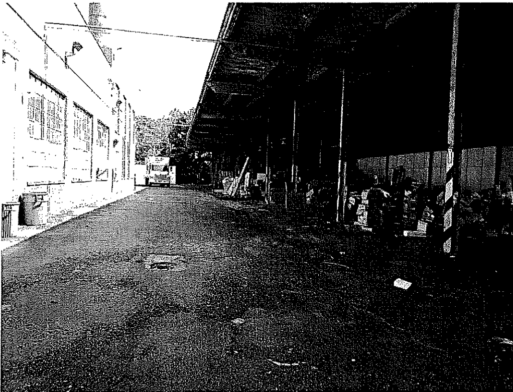
From north-west driveway looking south-east towards the back of the property.
