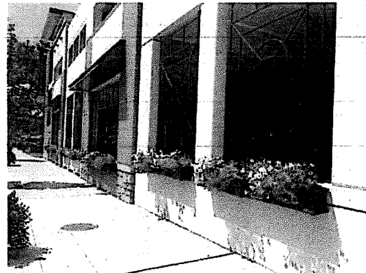
TimHaahs provided parking planning and design services for a 375-space parking facility to serve the Township of Millburn, NJ.
