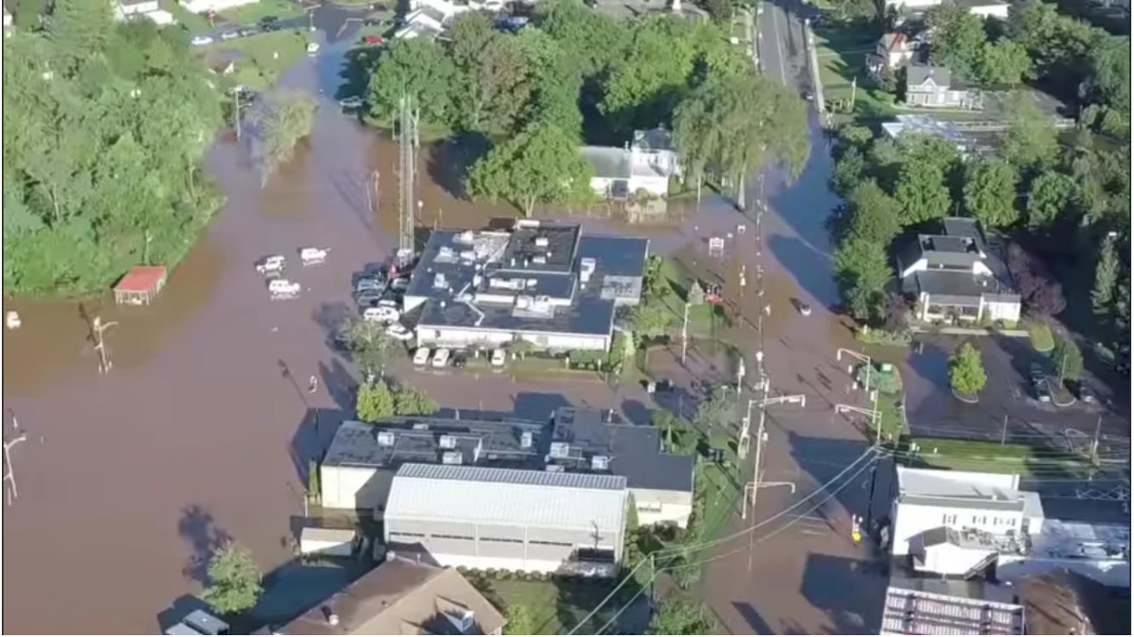
TROPICAL STORM IDA – SEPTEMBER 2, 2021; DAMAGED BASEMENT/LOST RECORDS
