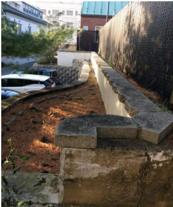
Photo B: Retaining Wall (Looking West)
