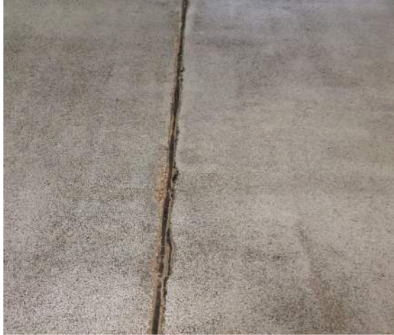
Photo #U1 – Joint at “T” Beams
