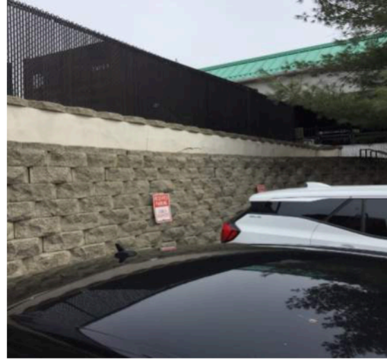
Photo #R2- Lower Modular Block Retaining Wall
