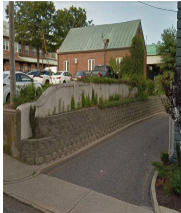
Photo C: Retaining Wall (Looking East)
