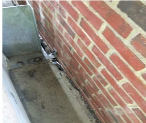
Photo #U2- Joint at Perimeter Slab & Walls
