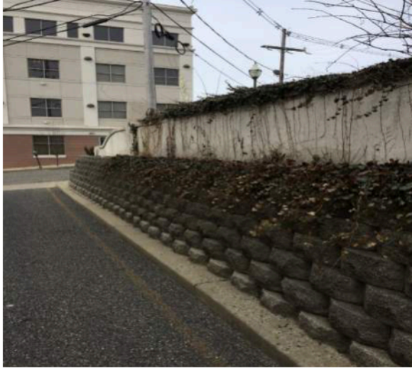
Photo #R1 – Two Tiered Retaining Wall
