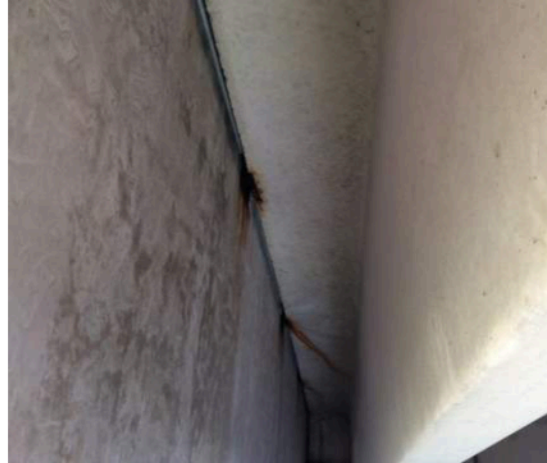
Photo #M2- Joint at Perimeter Slab & Walls
