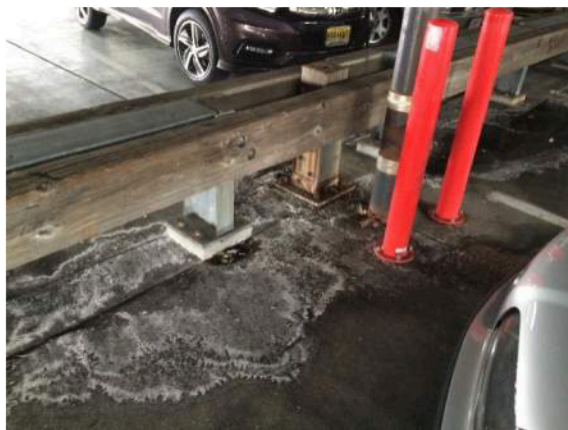
Photo #U3 – Joint at Center
