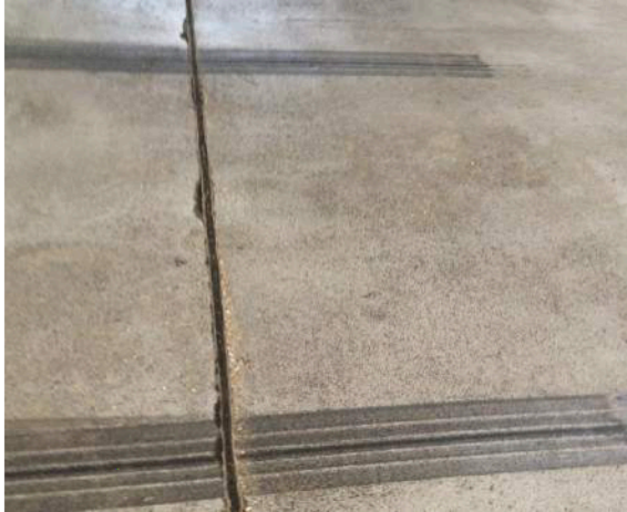
Photo #M1 – Joint at “T” Beams
