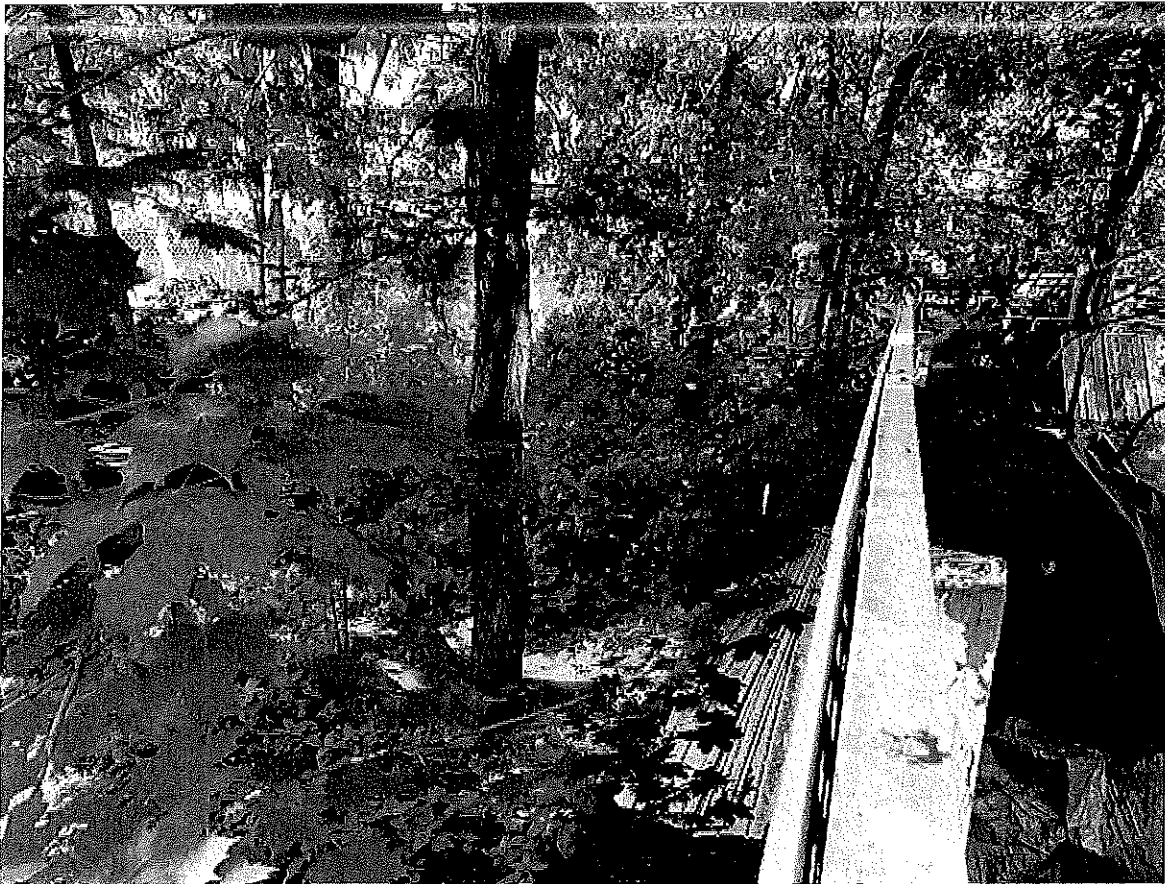
Photograph of overgrown brush and siding in the rear of 328 Harvard Ave
