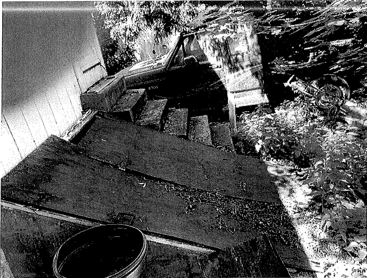
Photograph of Bilco Doors on rear of 328 Harvard Ave
