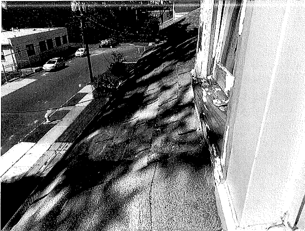
Photograph of roof in front of third floor window of 328 Harvard Ave
