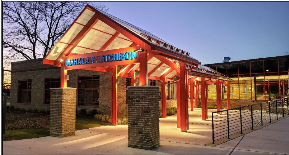
Mahala F. Atchison Elementary School (MFA)
