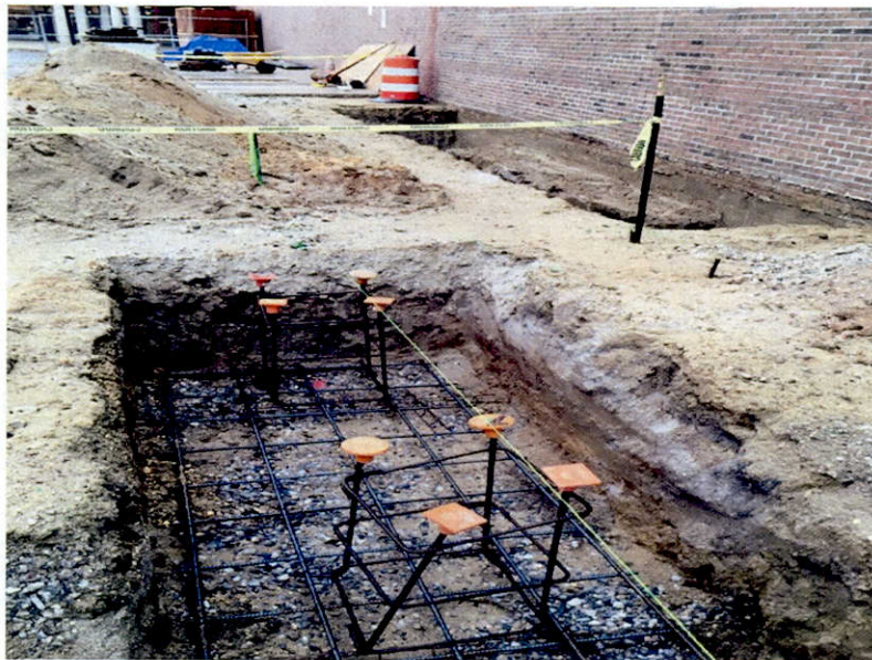
Attachment No. 4 Pier and Planter Footing Excavation
