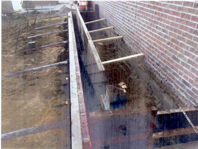
Attachment No. 3 Walls Prior to Concrete Placement
