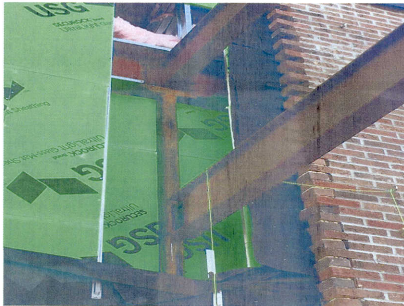
Attachment No. 2 New Framing To Existing Structure
