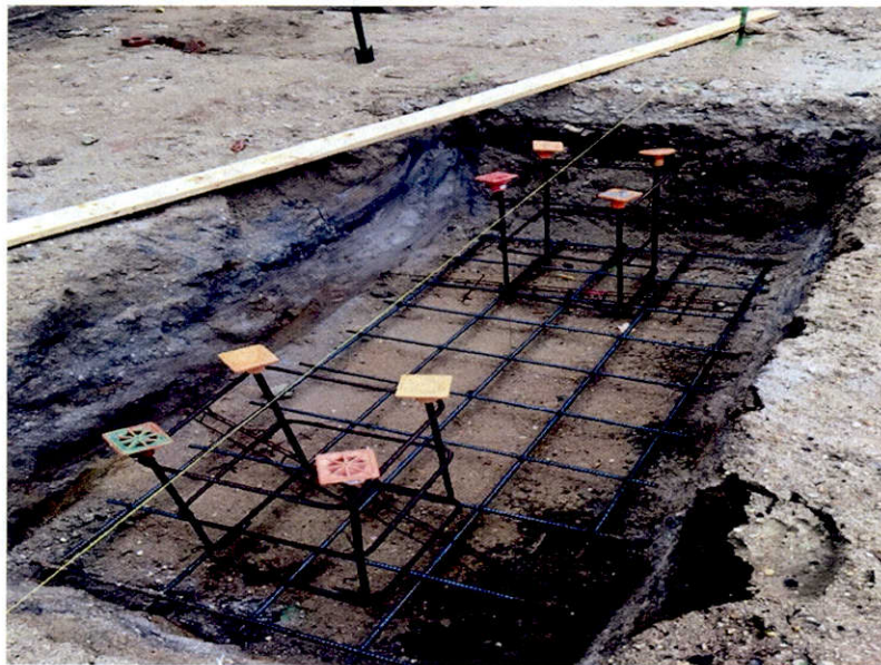
Attachment No. 2 Pier Footings
