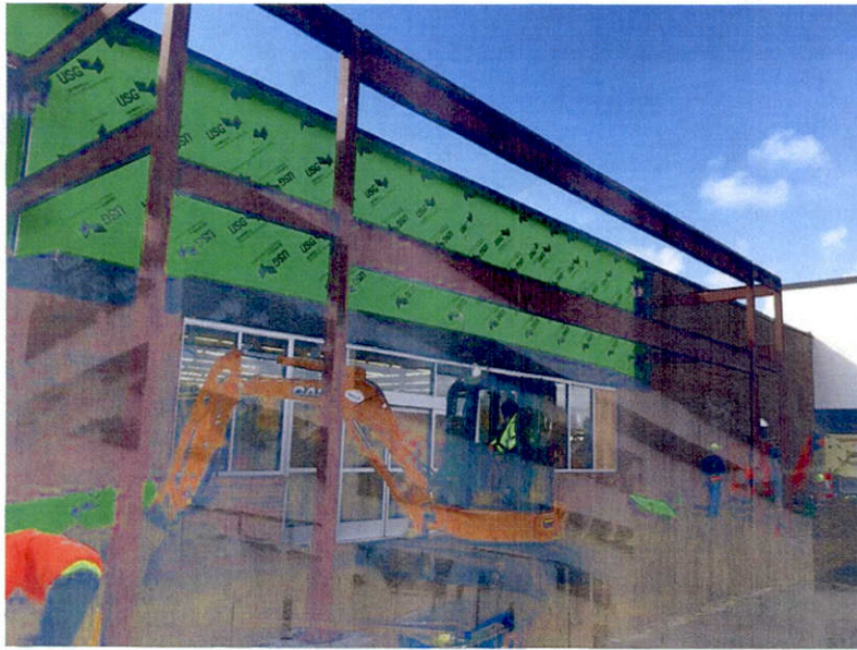
Attachment No. 1 Proposed Canopy Framing
