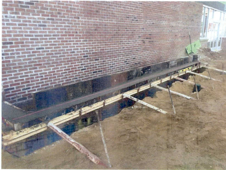
Attachment No. 5 Walls Post Concrete Placement
