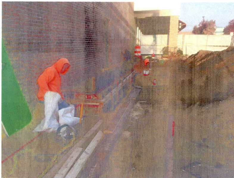
Attachment No. 4 Walls Prior to Concrete Placement
