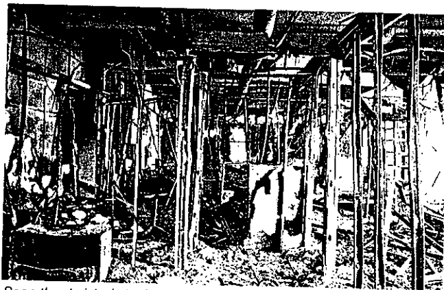
Seen thru twisted steel studs and total chaos, Monokote remains bonded to beams supporting concrete and steel floors.
