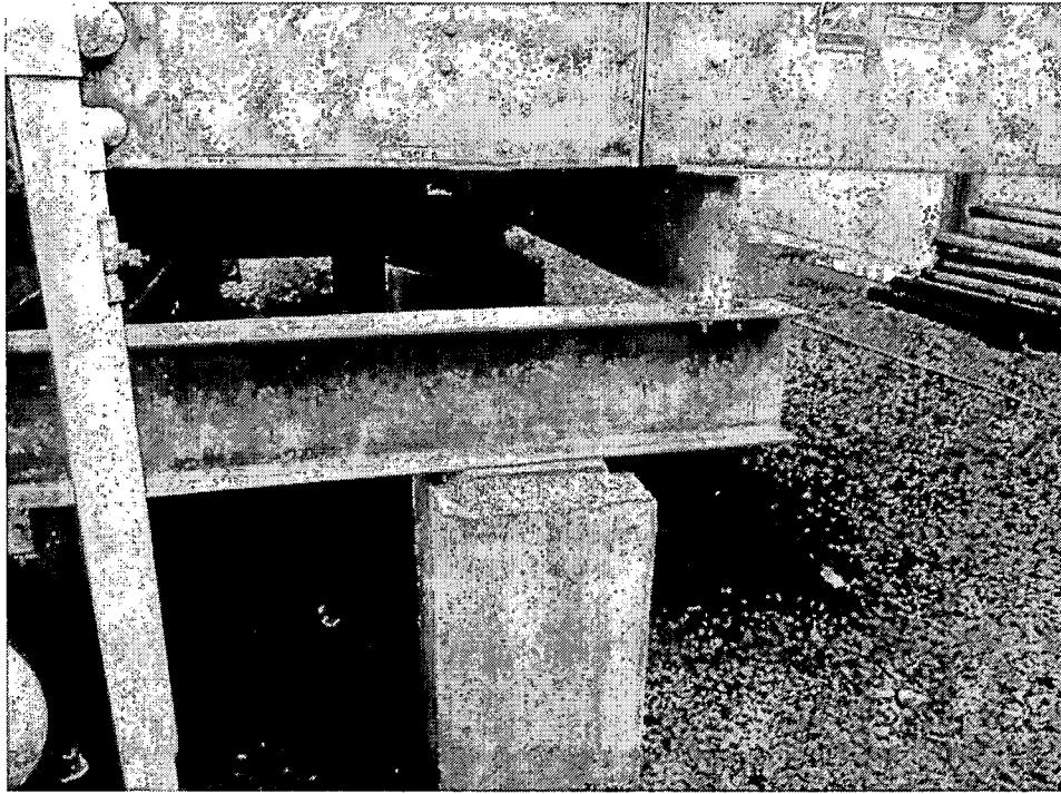
Figure 1 - Existing steel dunnage
