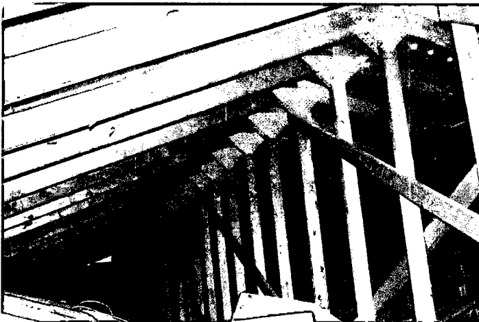
Photo 2 - Sloped bracing across center verticals.
