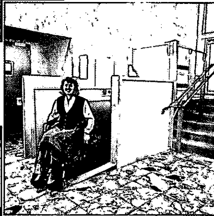
▲ Civic Center Lobby: An over-the-step bridge spans from the upper landing to the lift in this installation next to a staircase.
