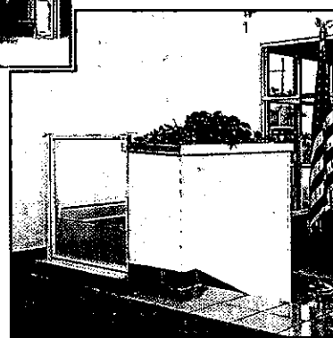
▲ Office Lobby: A clear acrylic panel in the top landing gate provides visibility.
