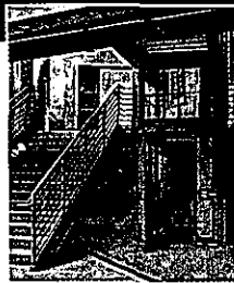
▲ Architectural Offices: Three-stop lift in a custom design, perforated stainless steel, I-beam enclosure provides access to lower level lobby and mezzanine offices.
