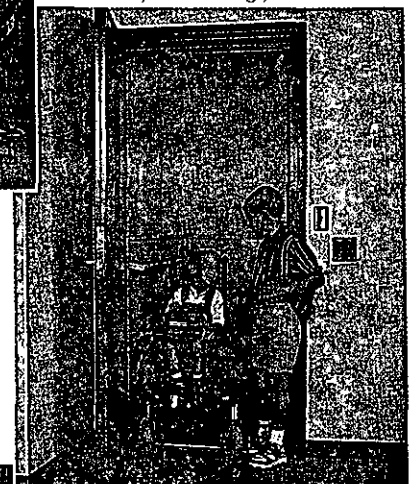
▼ Elementary School: A lift in a fully enclosed hoistway provides lower level access for a kindergartner.
