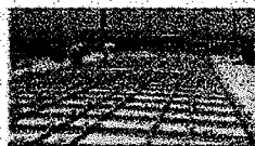
Interlocking grid design combined with Nexigen wind deflector reduces ballast to minimal or zero
