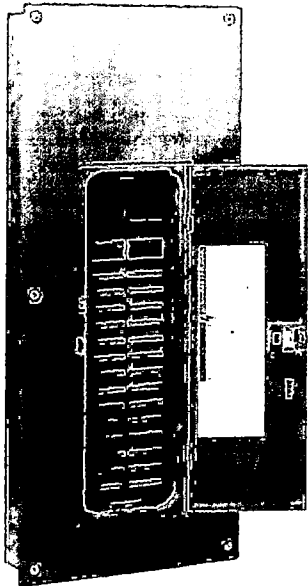
Main Service Panel
