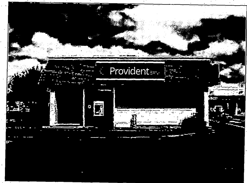
Existing Sign | 60 Square Feet
