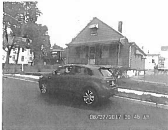
Photo# 5437, Replace side porch roof
