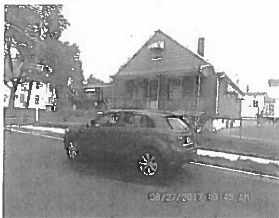
Photo# 5437, Replace side porch roof
