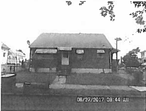
Photo# 5436, Repair or replace front steps
