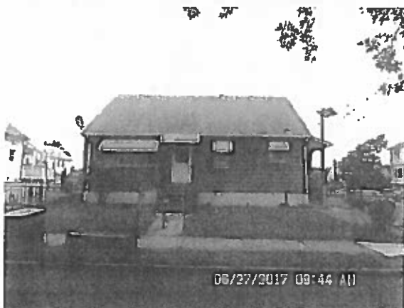
Photo# 5436, Repair or replace front steps
