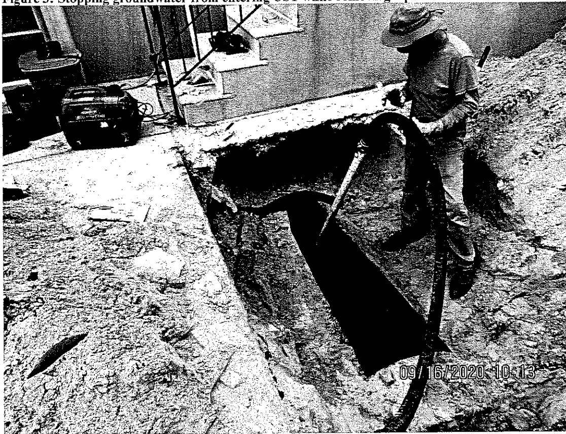
Figure 4: Approximately 60% of the UST is removed - no exterior staining
