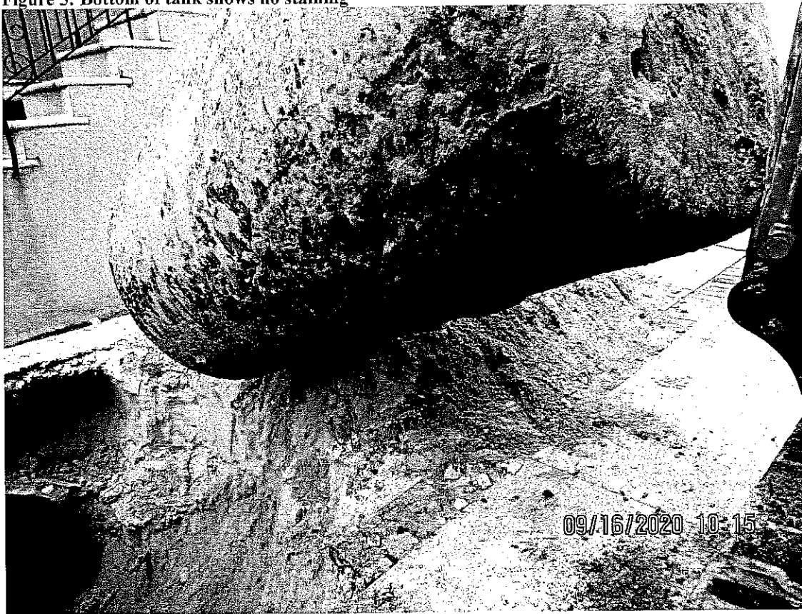
Figure 6: Open excavation shows no staining - sampling points shown
