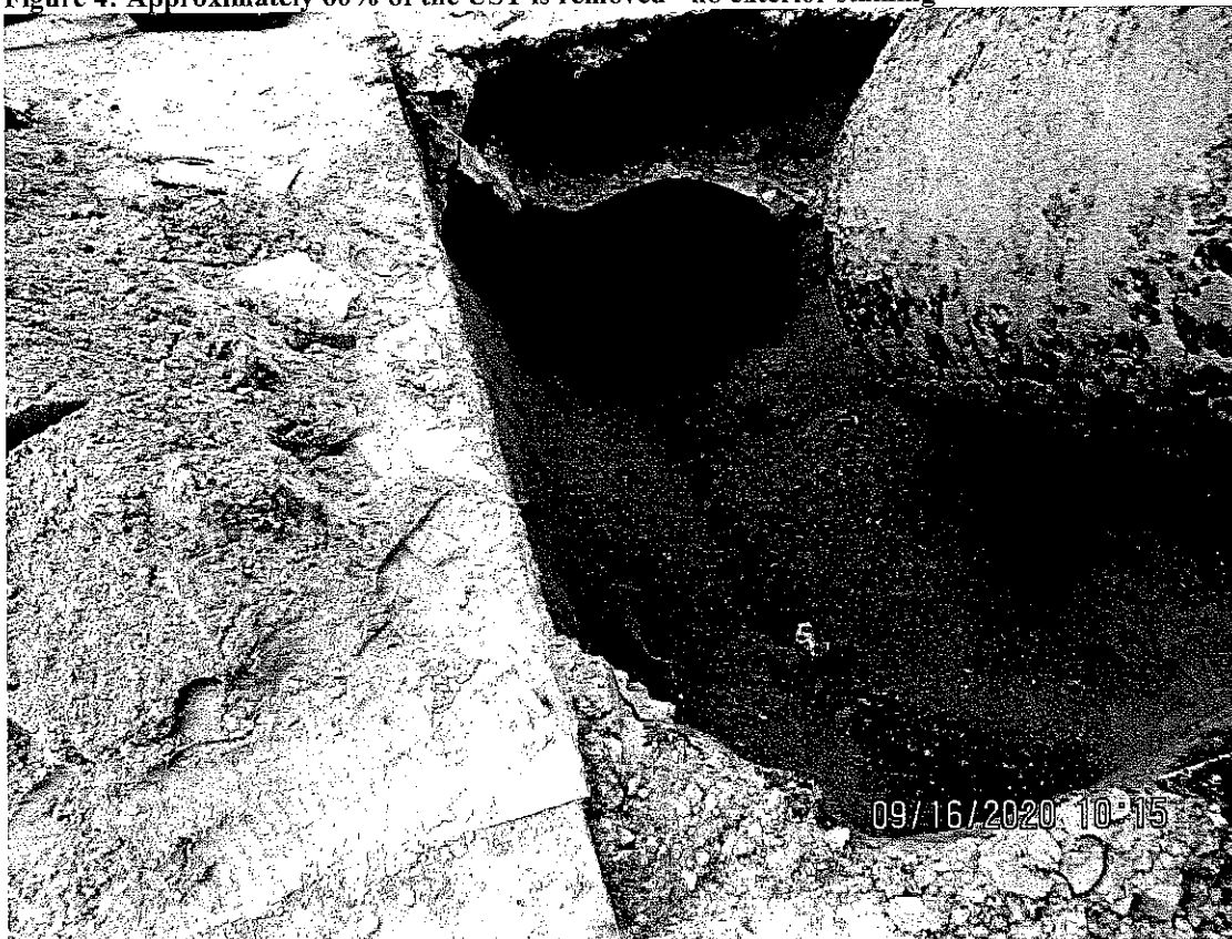
Figure 4: Approximately 60% of the UST is removed - no exterior staining
