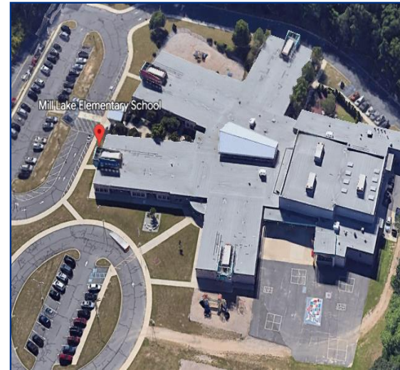
ROOFING REPAIR / REPLACEMENT
