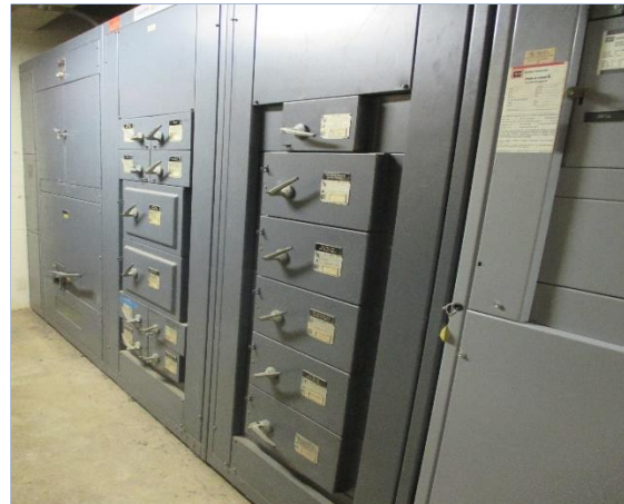
ELECTRICAL INFRASTRUCTURE UPGRADES
