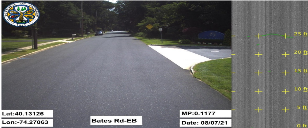
a) Bates Road (Eastbound Direction)
