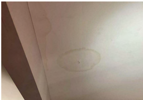
69156, Water damage
