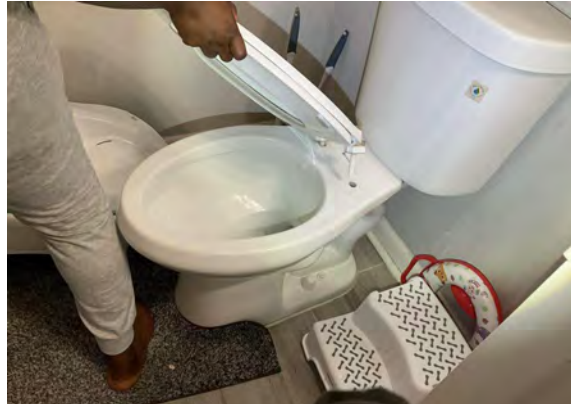
42027, Broken toilet seat
