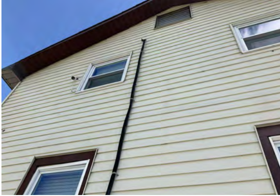
42034, HVAC in attic
