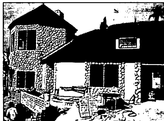
WHITEWATER RIVER ROCK —is applied with ordinary Portland cement mortar.
