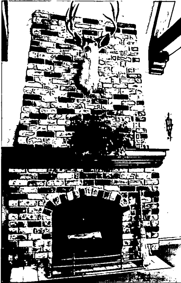
OLD USED —Right-angle corner pieces insure full thickness appearance.
