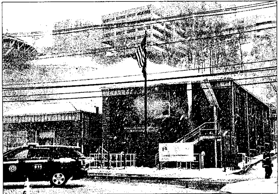
The North Hudson Regional Fire and Rescue successfully doused a 4 alarm fire at the Woodcliff Treatment Plant March 21. See briefs for more information. (Photo credit: Art Schwartz)
