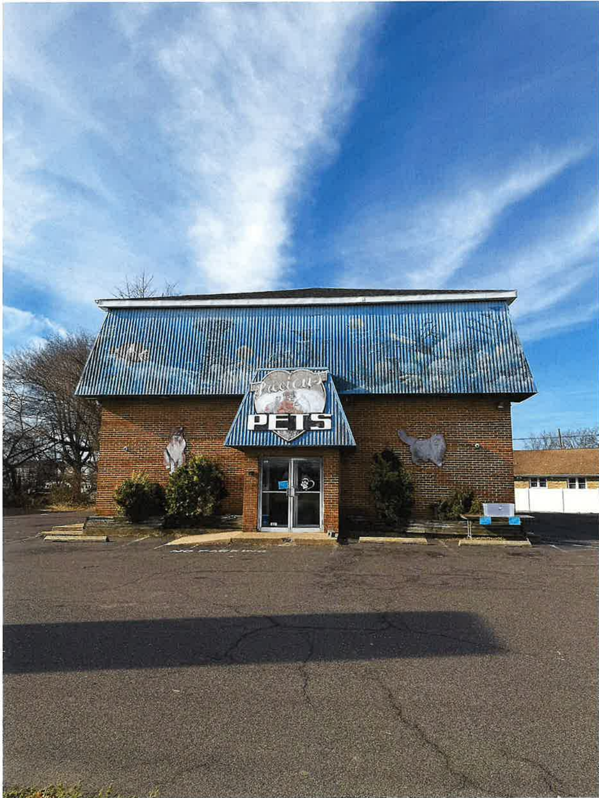
Figure 2 - View looking Northwest at front of existing building to remain.
