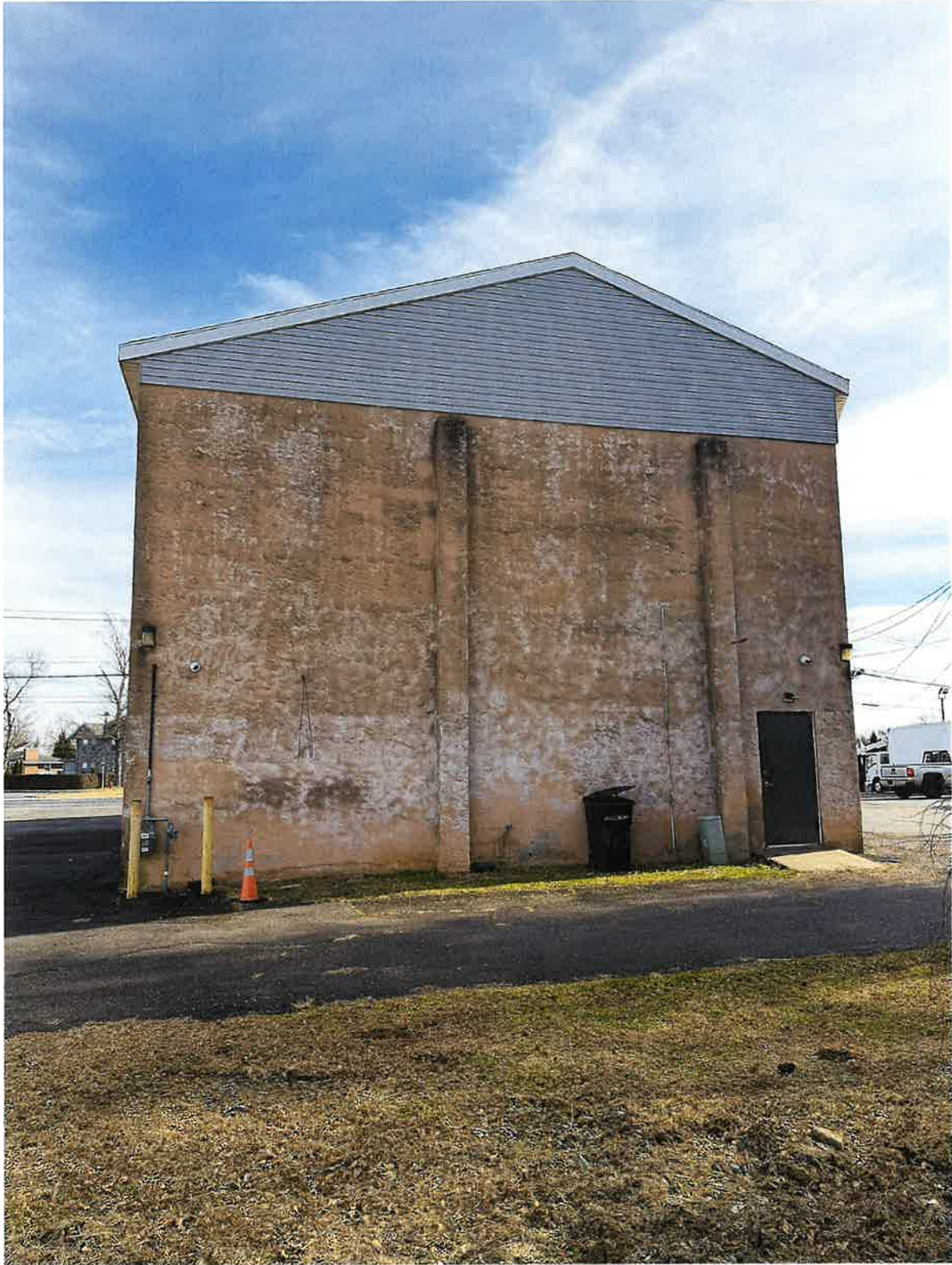
Figure 5 - View looking Southeast at rear of existing building to remain.
