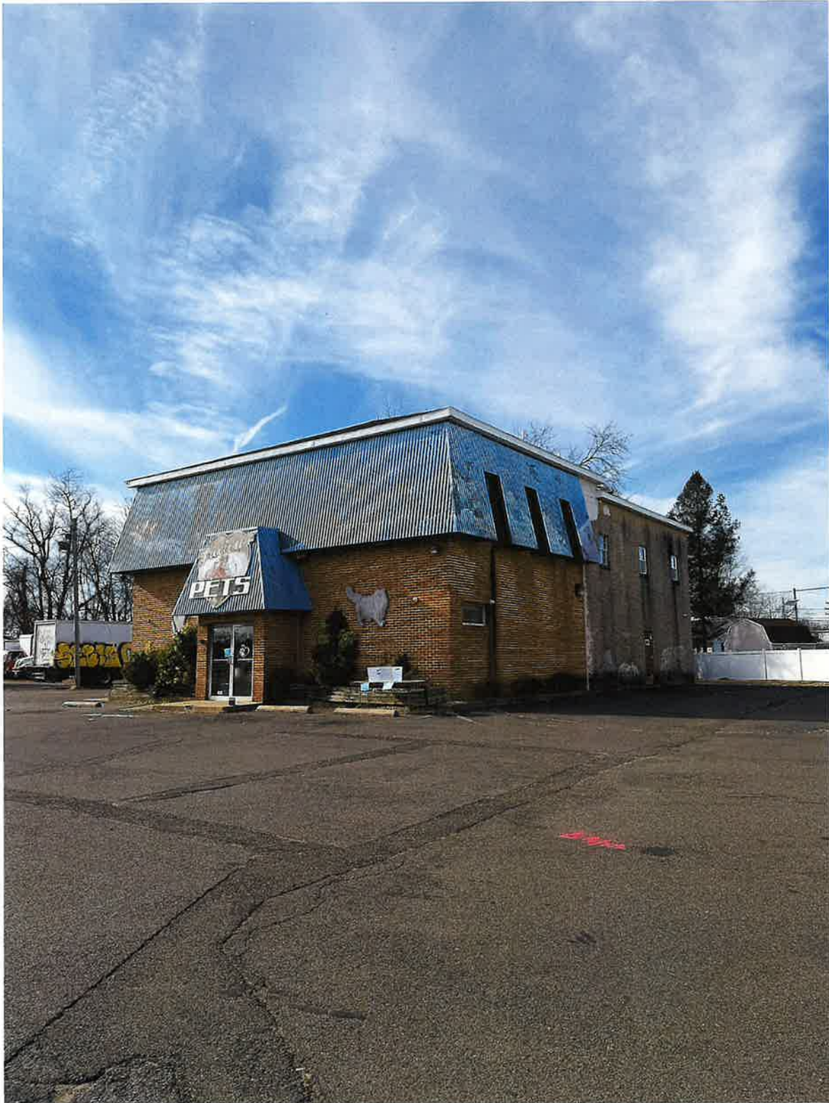
Figure 3 - View looking West at front of existing building to remain.
