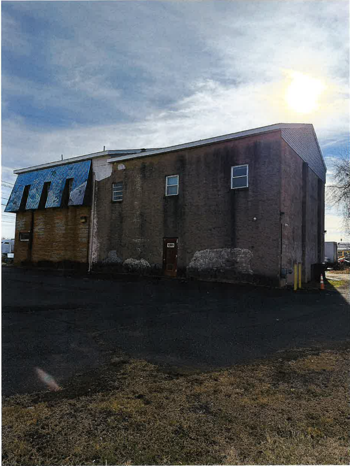
Figure 4 - View looking South at existing building to remain.
