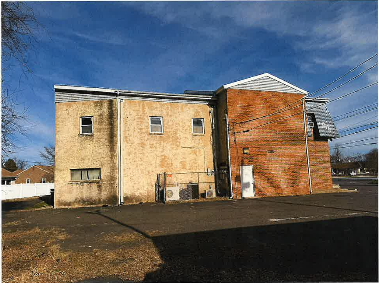
Figure 6 - View looking Northeast at existing building to remain.
