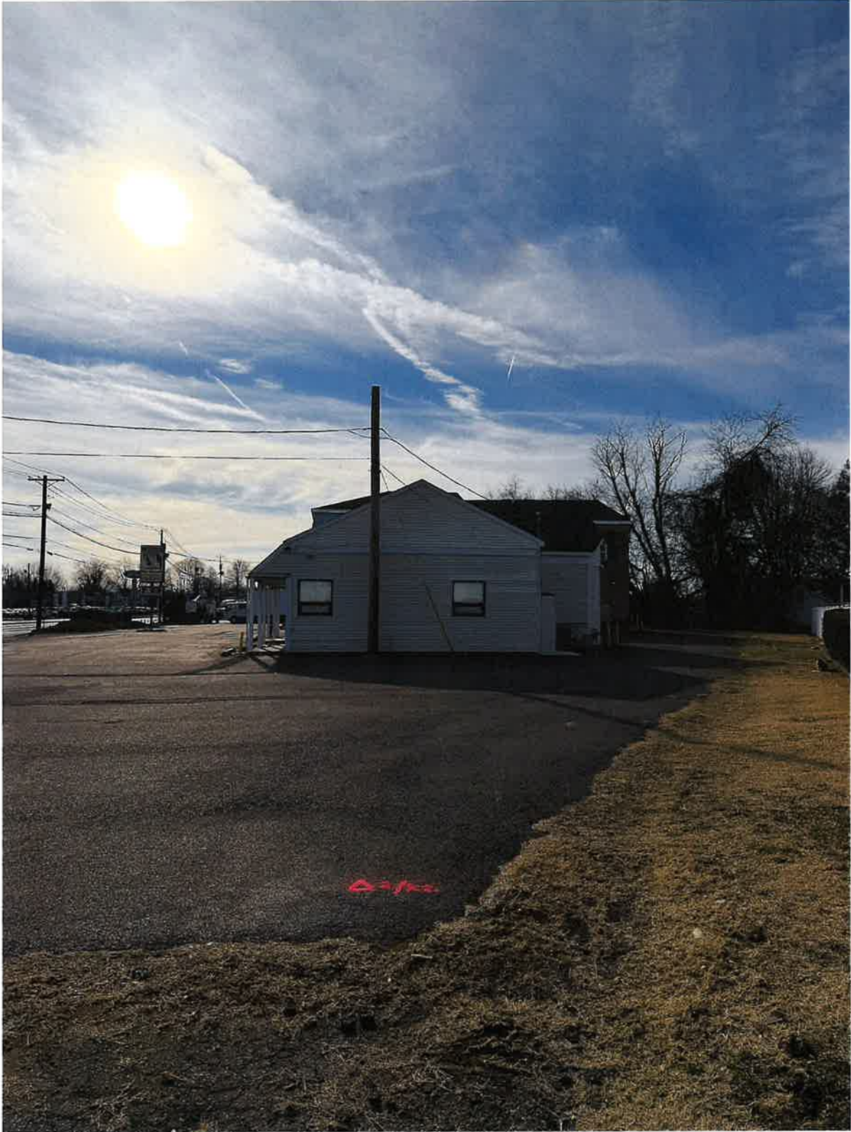
Figure 9 - View looking Southwest at existing building to be removed.
