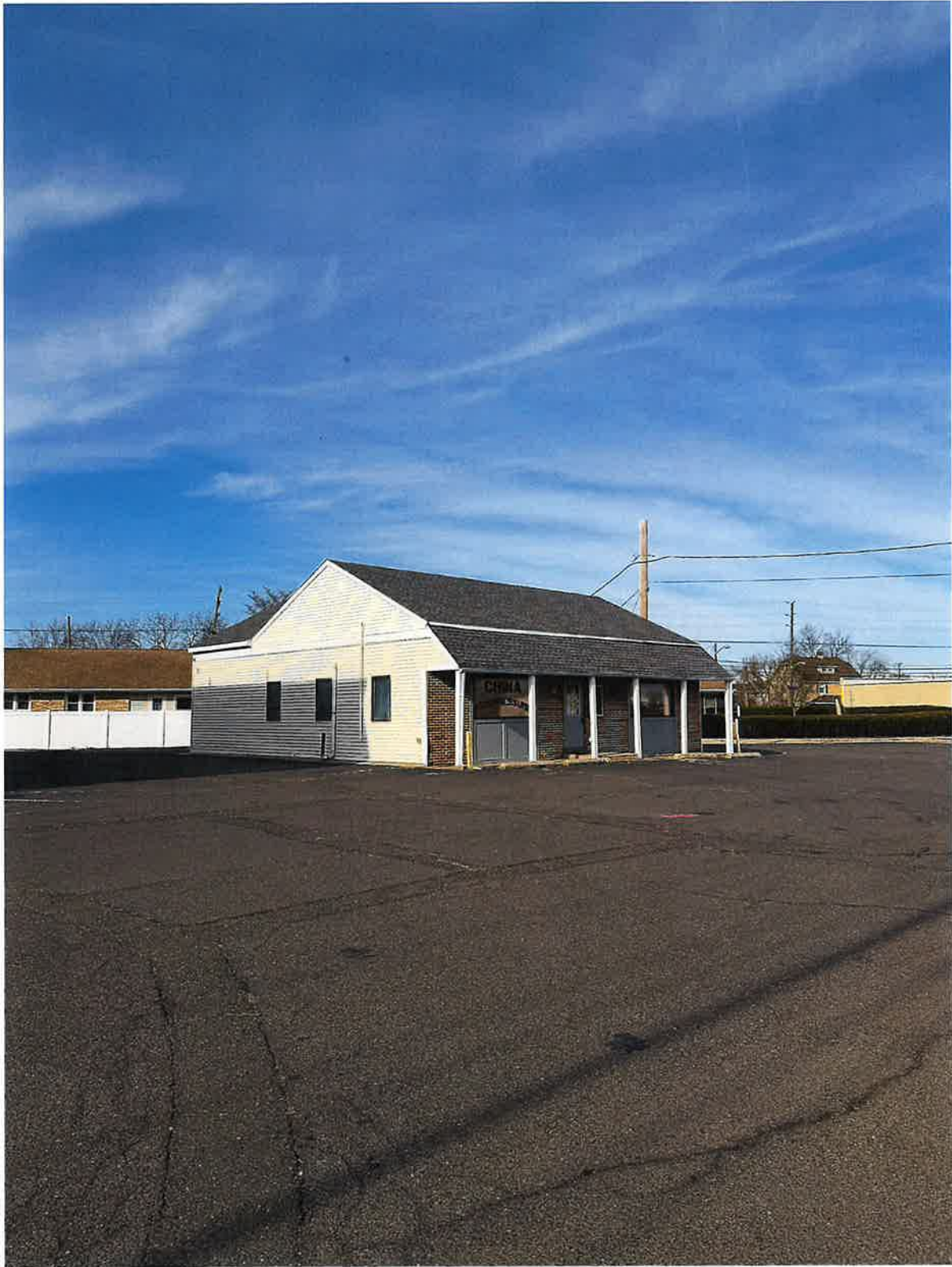
Figure 7 - View looking North at existing building to be removed.
