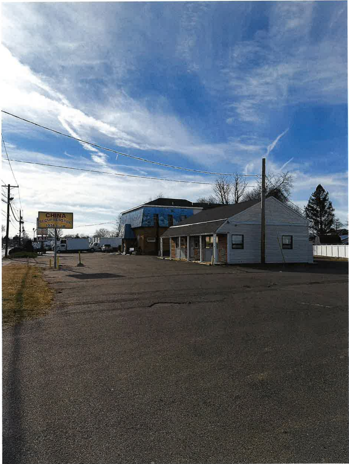
Figure 8 - View looking West at existing buildings on site.
