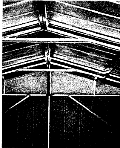
Steel Reinforced Trusses!
