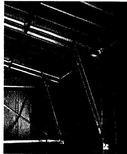
Steel Reinforced Trusses!
