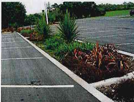
Rain Garden in Parking Lot
