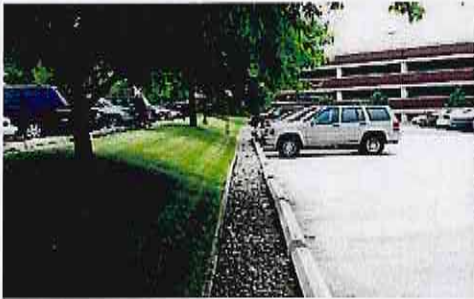
Infiltration beds in a parking lot
