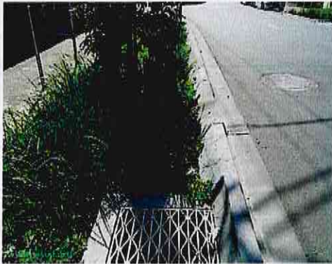
Bioretention swale retro-fit to roadway
