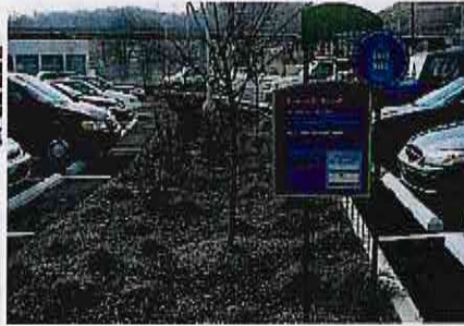
Bioretention swale in a parking area
