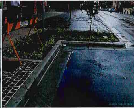
Street tree stormwater treatment retro-fit
