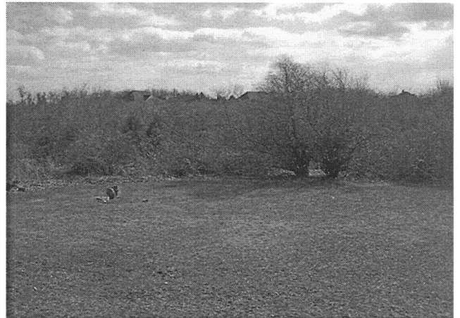
Heavy vegetation on absorption area.
