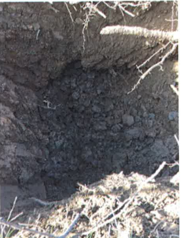
Dry gravel in the disposal area.
