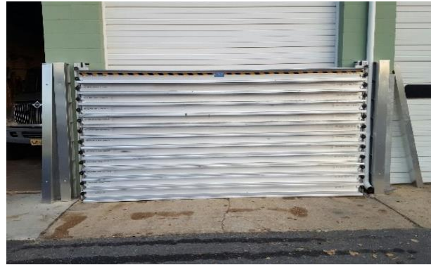
Community Action #42_4: HMGP-funded flood-proofed doors at Rumson's DPW building, which experienced 4 feet of water during Superstorm Sandy. Photo courtesy of Borough of Rumson.
