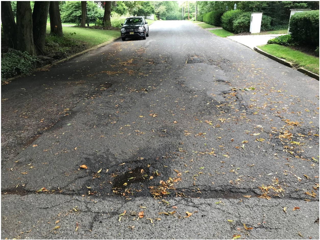
Cooney Terrace at Hance Road
