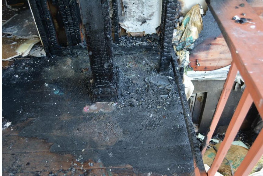
Area cleared of debris
