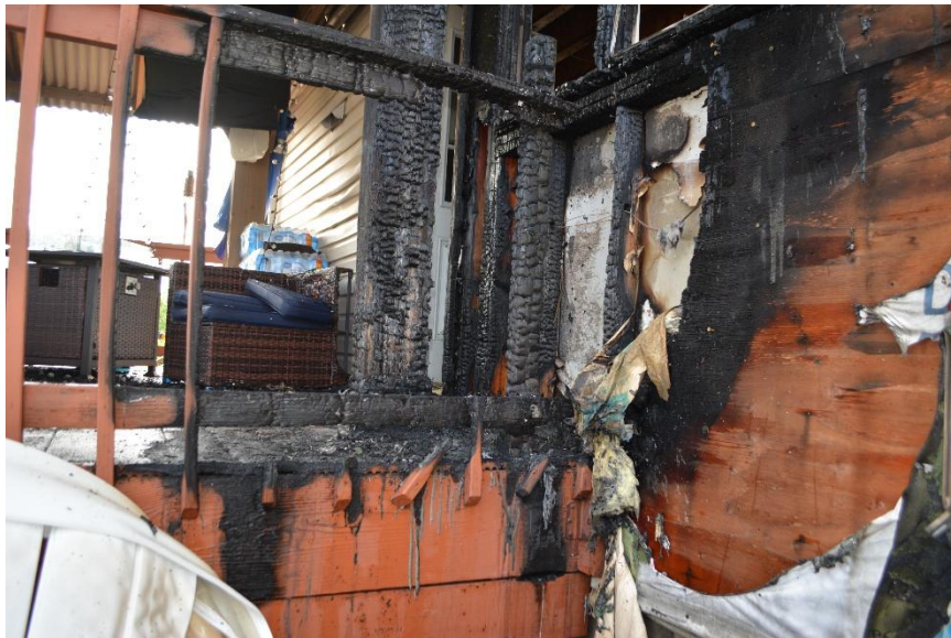
Side view of the deck
