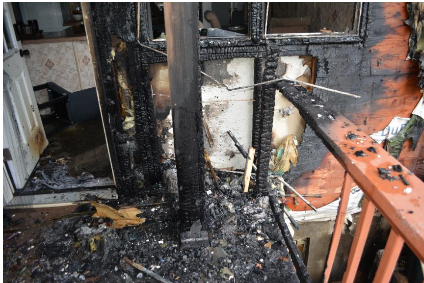
Close up view of the right rear side of the deck
