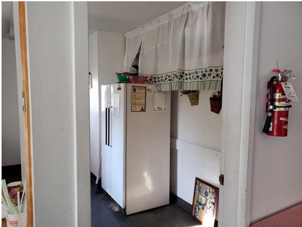
Existing doorway and narrow entrance area in kitchen area.
