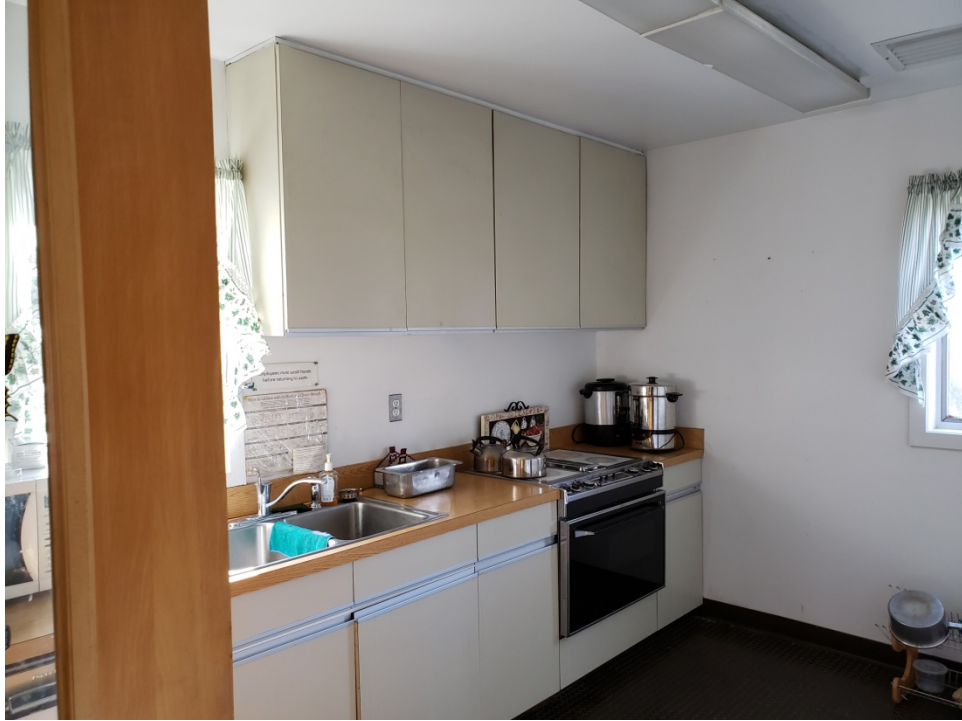
Existing kitchen area.
