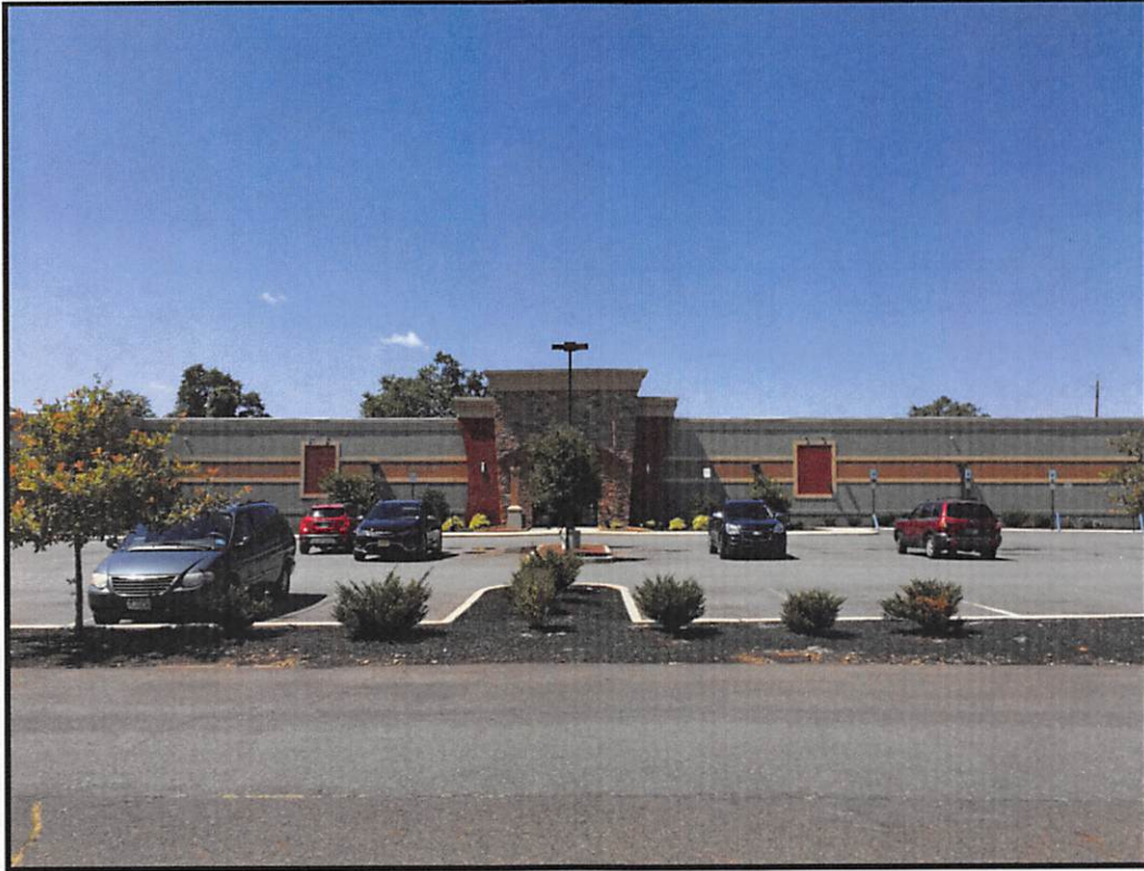
Photo 1: View of the bowling alley.
