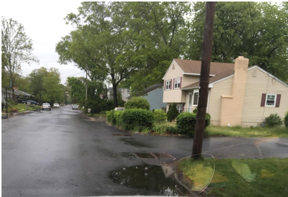
Anchor Avenue – Inlet E-2
