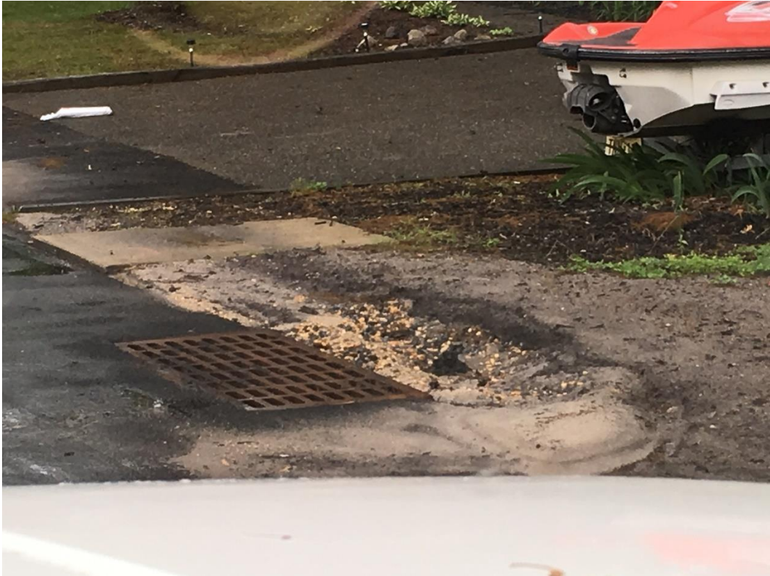
Anchor Avenue – Inlet A-6
