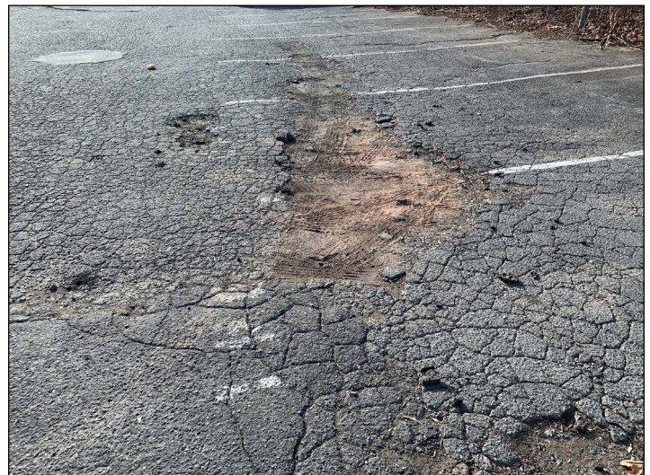
Figure 4: Deteriorated or missing pavement in parking spaces on Lot 28.
