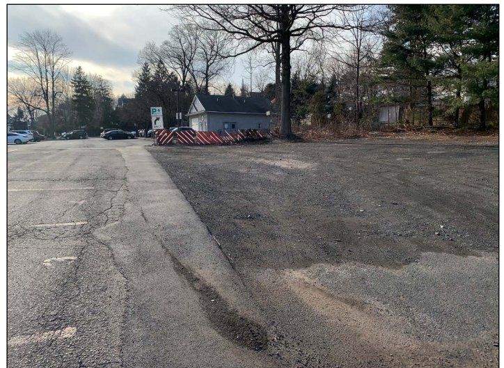
Figure 10: Uneven parking and circulation surfaces at southwest corner of Lot 30.
