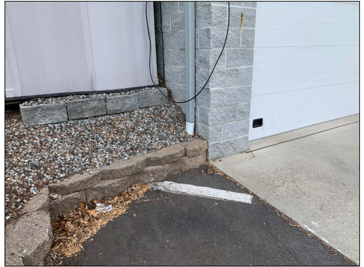
Figure 4: Downspout from fire station building, leading to storm sewer system.
