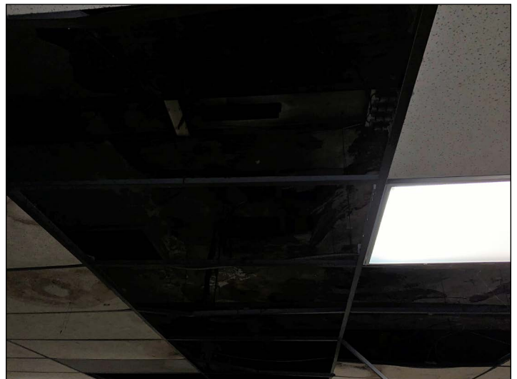
Figure 8: Failed ceiling and roof.
