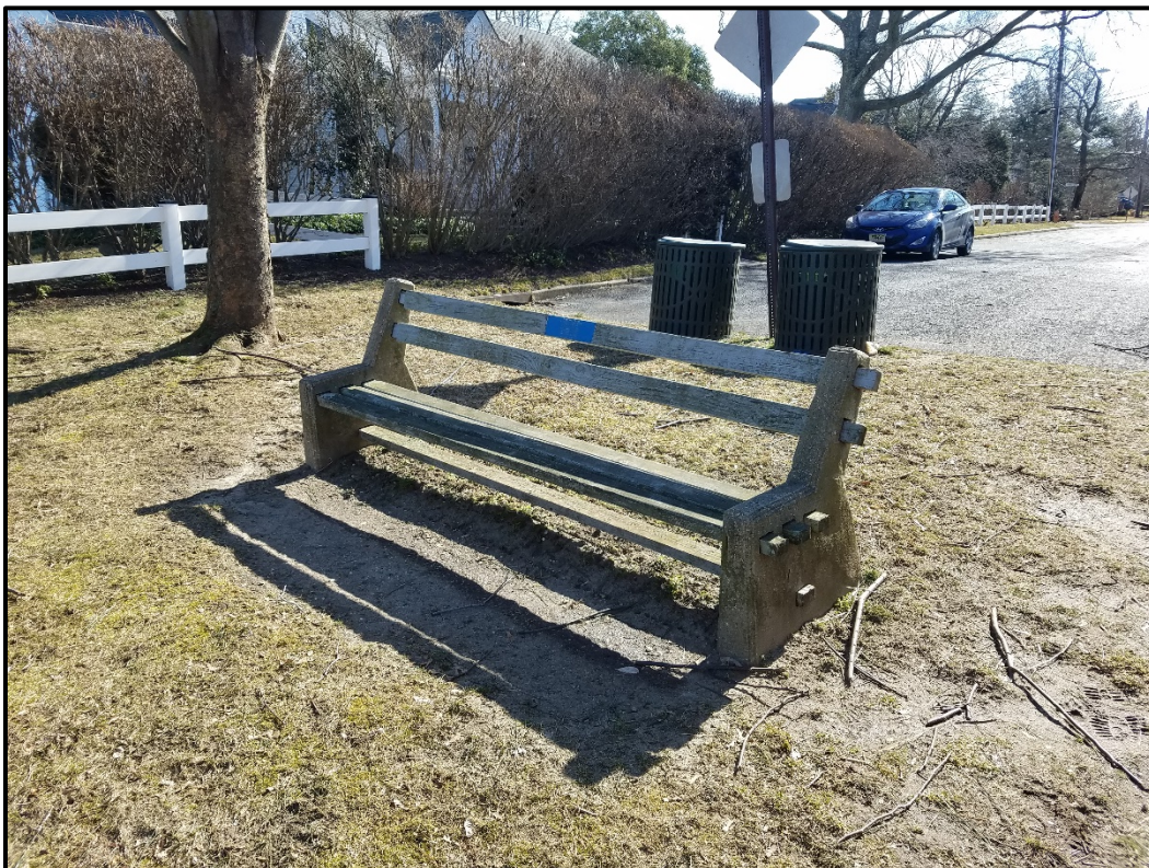
Photo view 4. Easterly view of parking and road end and benches to be removed and repaired.
