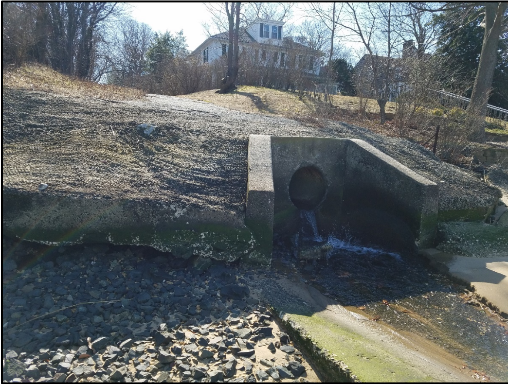
Photo view 5. Southwesterly view of adjoining residential property, slope and drain.
