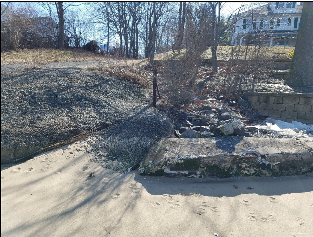
Photo view 6. Southeasterly view of road from beach and residential properties.
