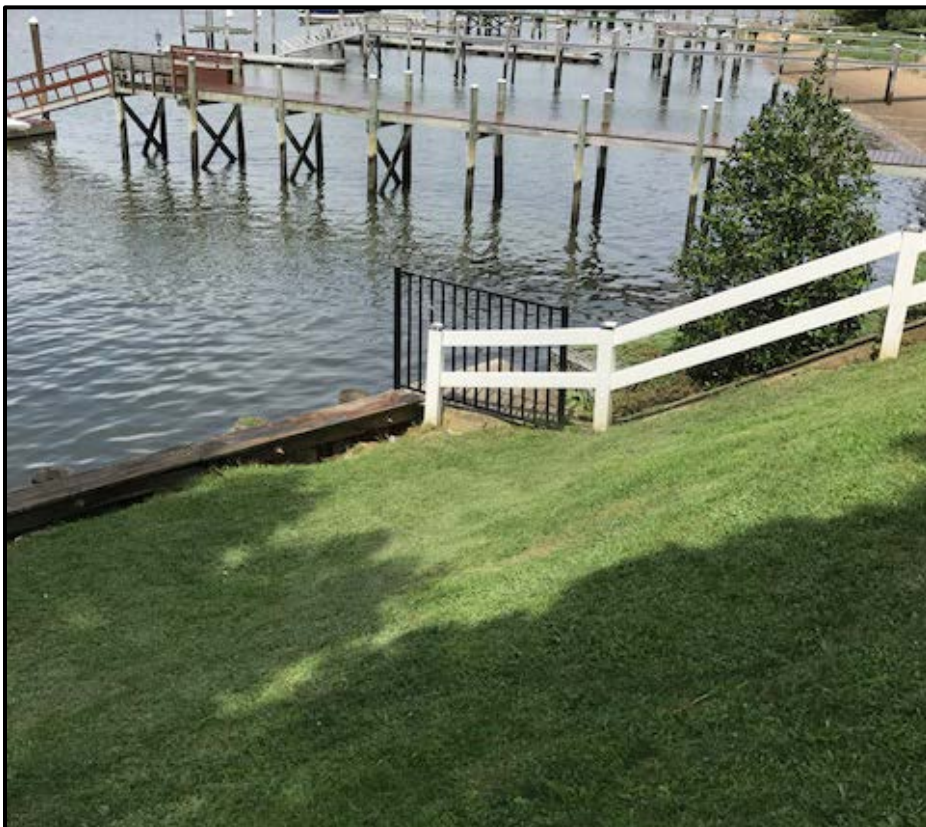
Photo view 6. Northeasterly view of slope and bulkhead.
