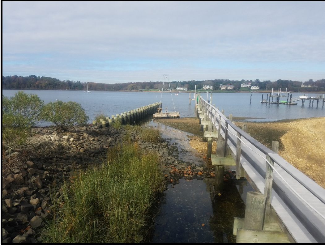
Photo view 3. Northwesterly view of existing bulkhead/breakwater.
