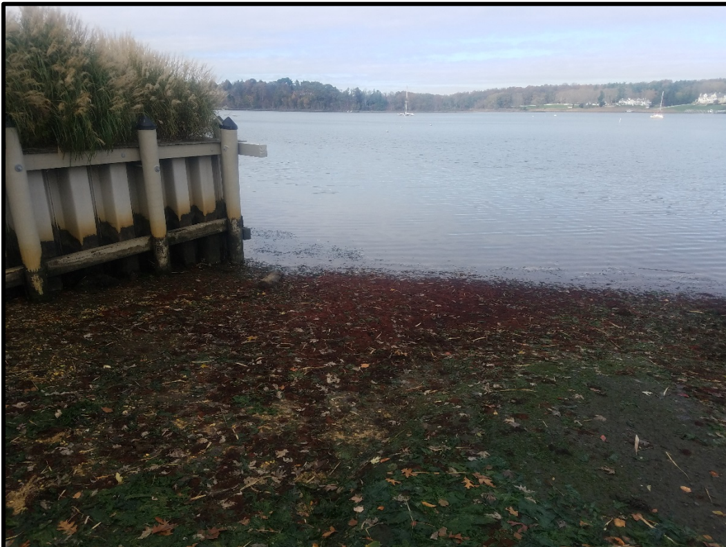
Photo view 4. Northerly view of boat ramp and adjoining bulkhead to the west.
