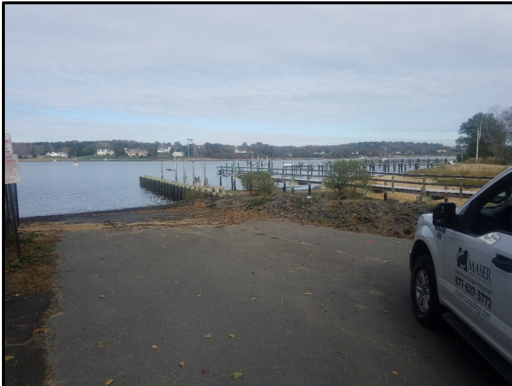
Photo view 2. Northeasterly view of existing boat ramp and bulkhead.
