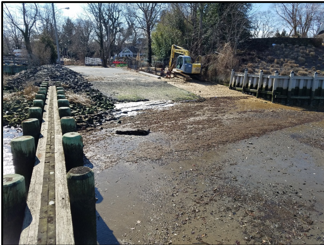
Photo view 6. Southwesterly view of boat ramp and adjoining bulkhead.
