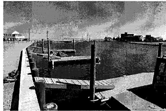
View of Bulkhead/Floating Docks Along Creek (Photo Taken on March 17, 2017)
