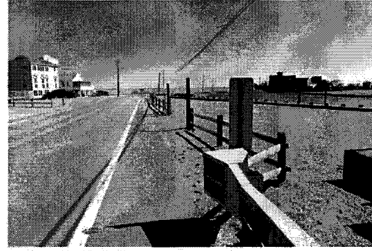
Southeast View Along Cedar Run Dock Road (Photo Taken on March 17, 2017)
