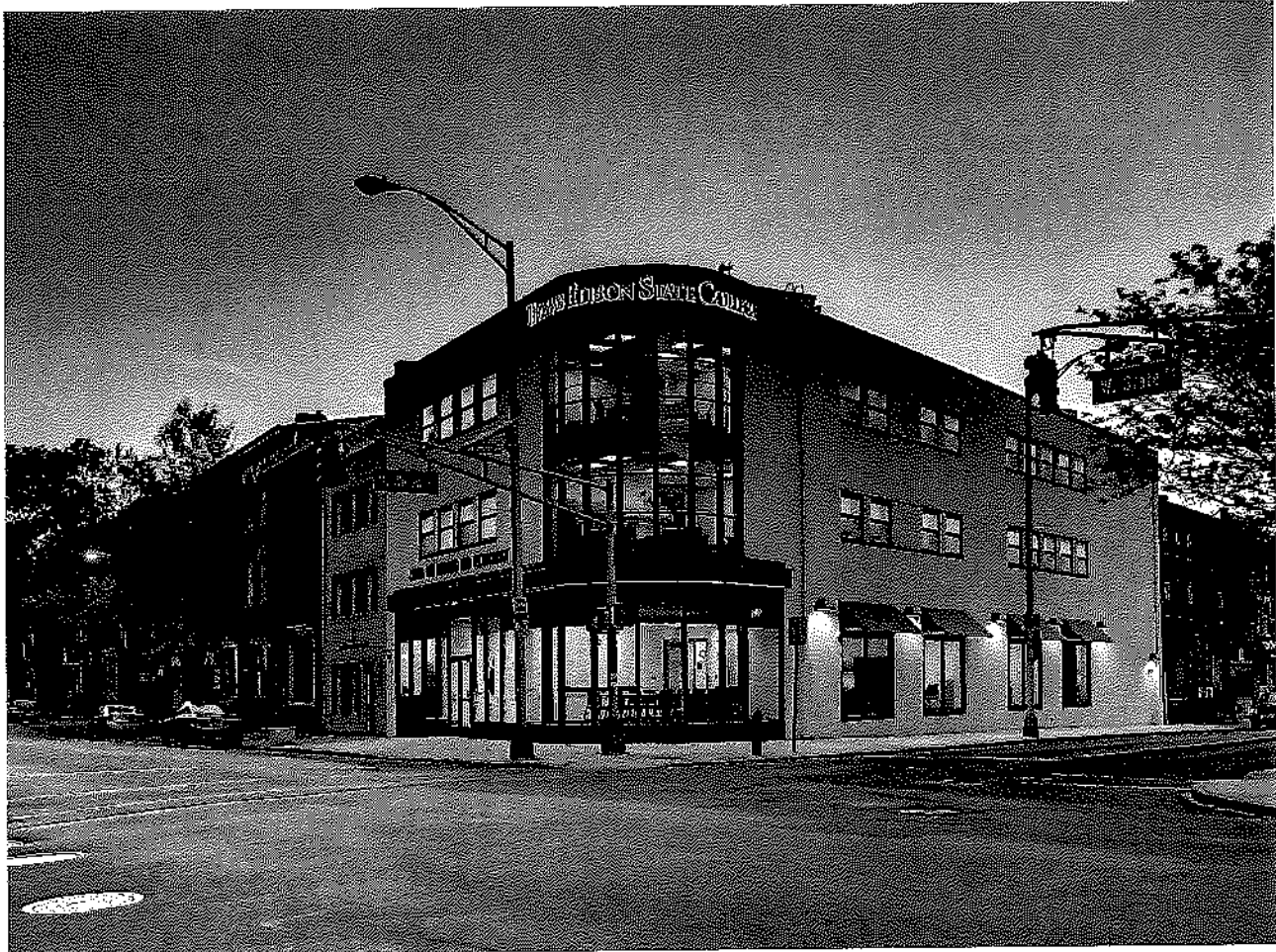
View from State Street
