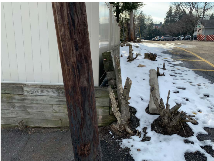
Figure 9: Unstable wooden wall along property line between Lots 30 and 31.
