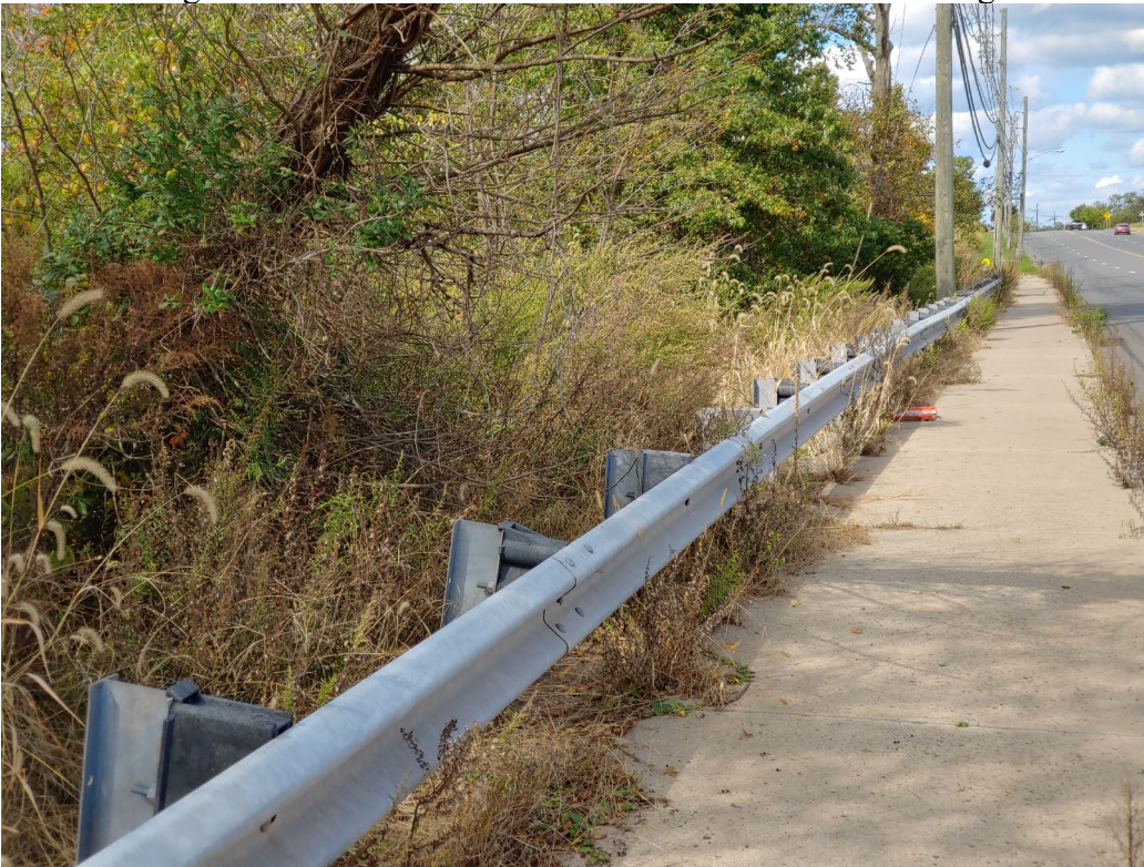
(Street view of culvert on Lot 12)
