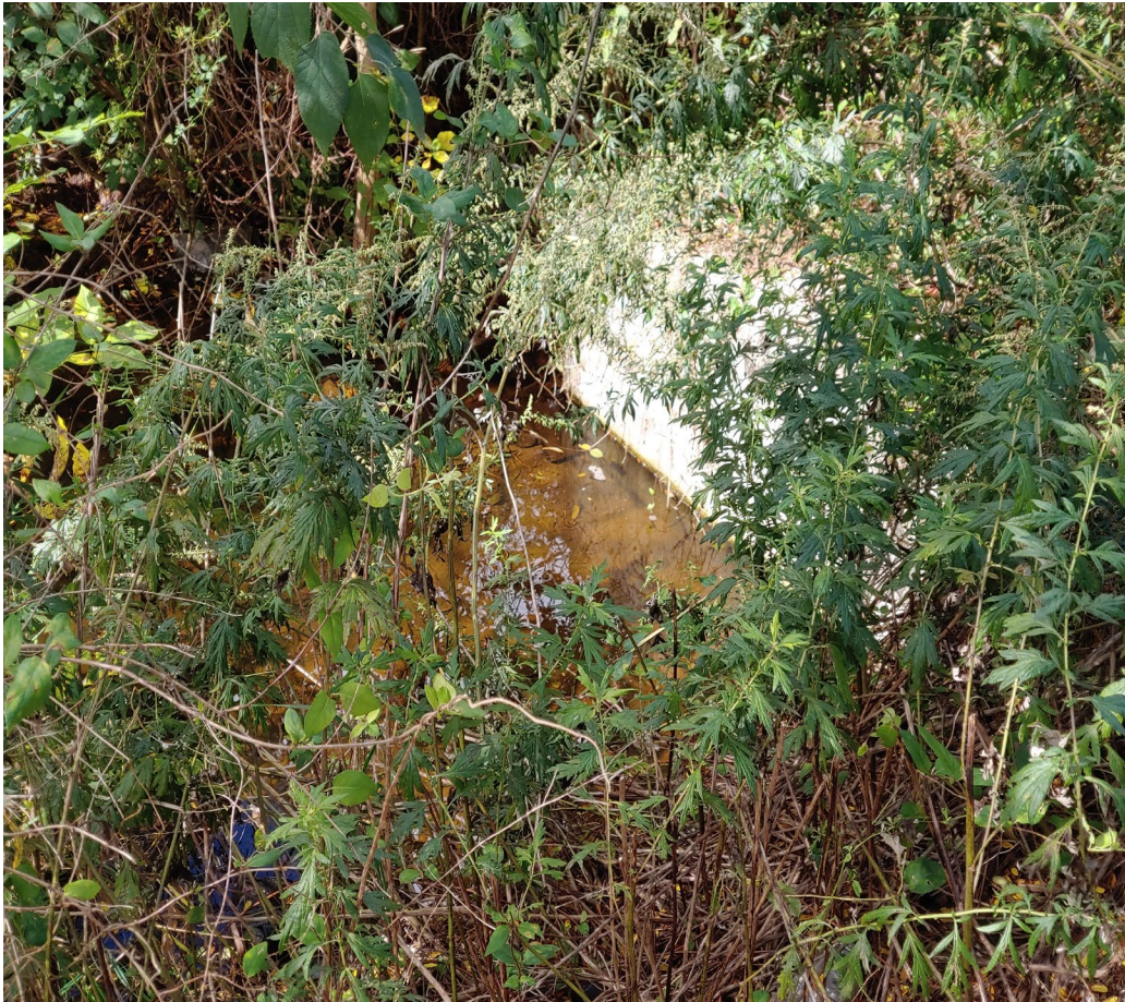
(Water flowing under a culvert from Lot 12 underneath South Washington Avenue)
