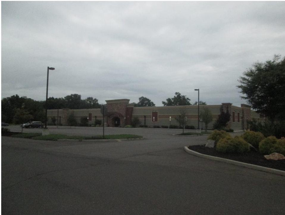
Remainder View Looking Southwest
