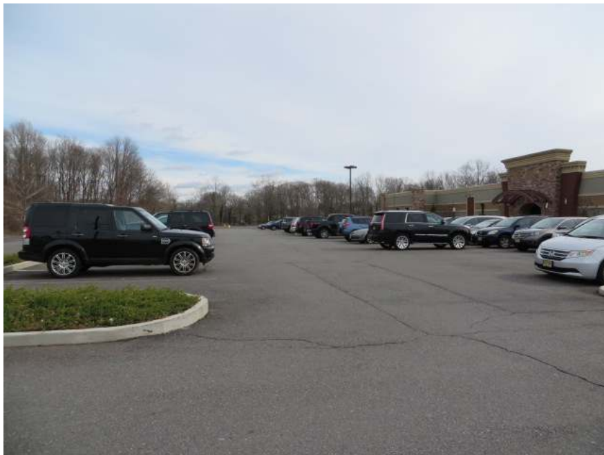
Existing Parking Lot
