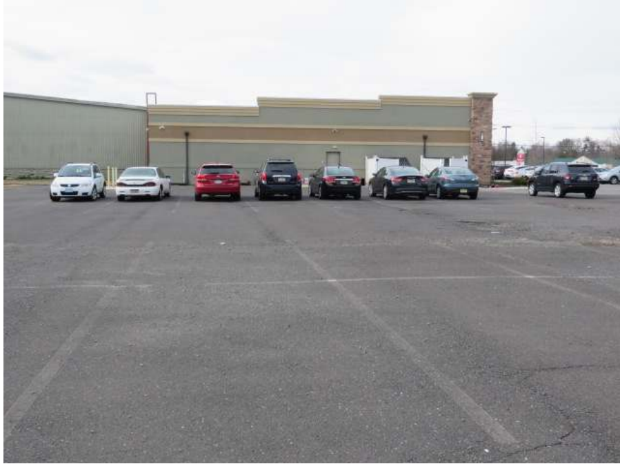
Rear Parking Lot – Partial Acquisition Area Extended Stay Area
