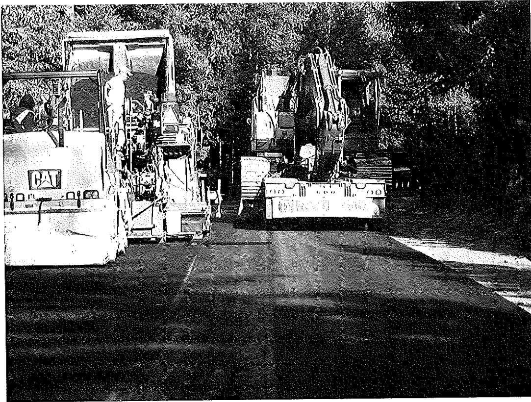
Photo credit: Independent Highway District, ID. Pictured are pavers installing divots for Recessed Lane Indicators.
