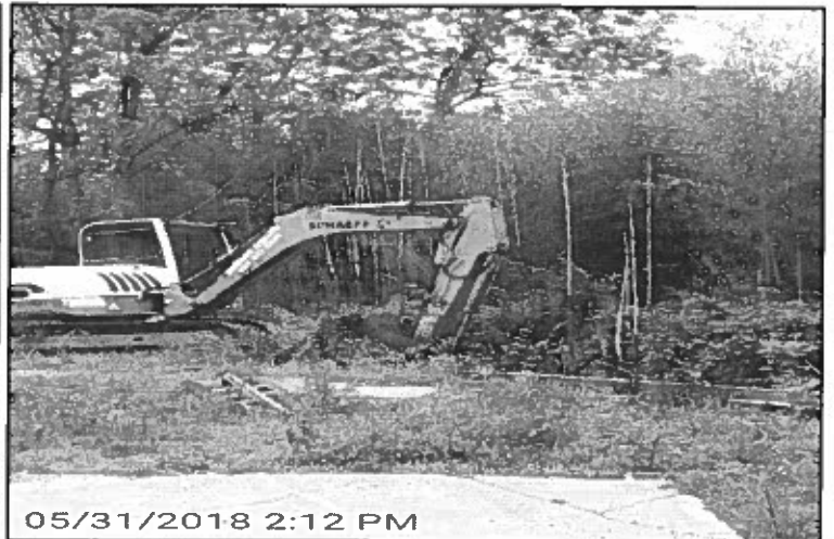
Description: SDLMobile - Inspection Photo
