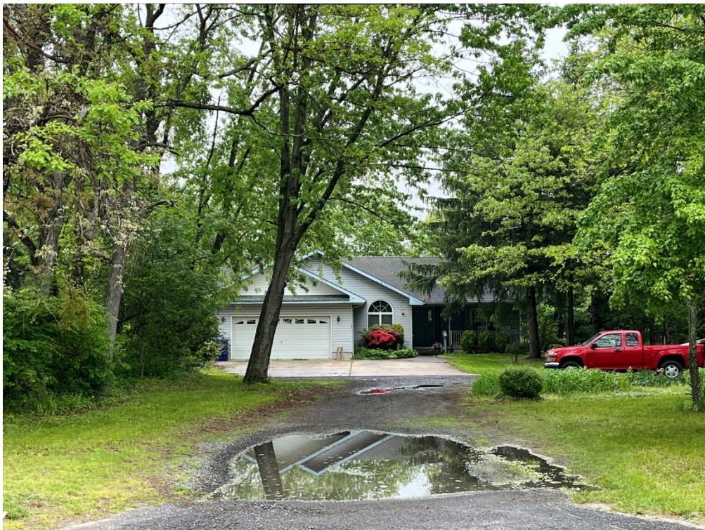
Existing residential dwelling to be subdivided off
