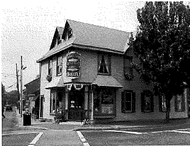
Robin's Nest Restaurant, Mount Holly, NJ JoAnn Weininger at 609-267-8600 Fully reinforced system on mid-1800s standing seam roof
